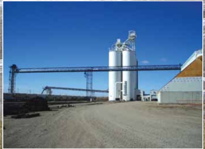
Long-Span and Walk-Through Truss Conveyors.
